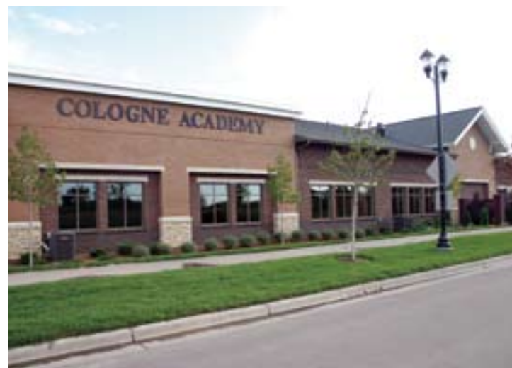
The new 16,000-square-foot Cologne Academy is located next to the city's community center.
