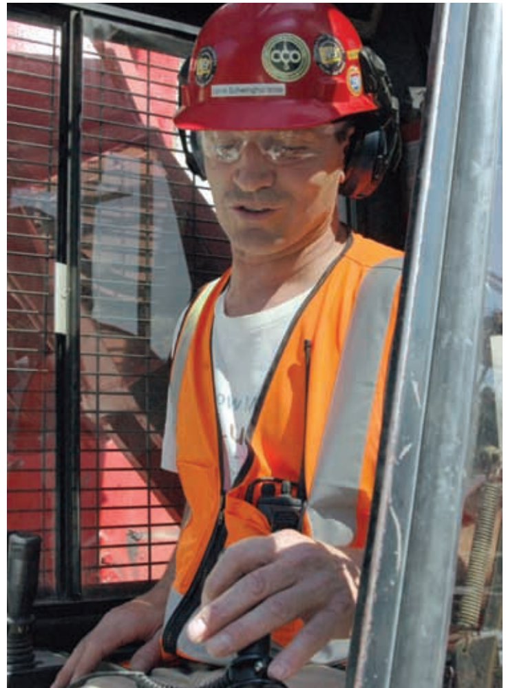
Loren Schwinghammer of Cologne is a crane operator on the I-35W bridge construction project in Minneapolis. He operates cranes weighing up to 275 tons, with 300-foot booms. Three of his 14 brothers are also working on the project.
